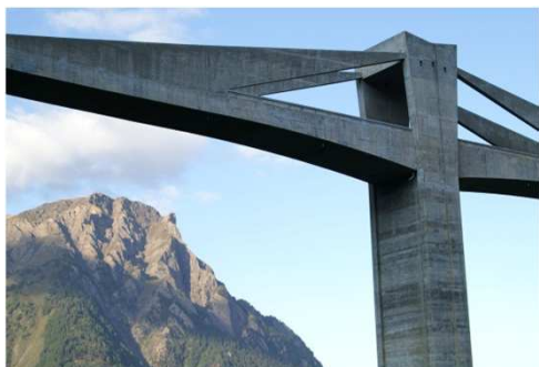
Figure 3: Ganter bridge, Switzerland
