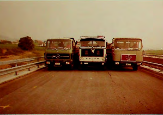
Empa report 41'002 - Load Test on Swiss a bridge (1979 )
