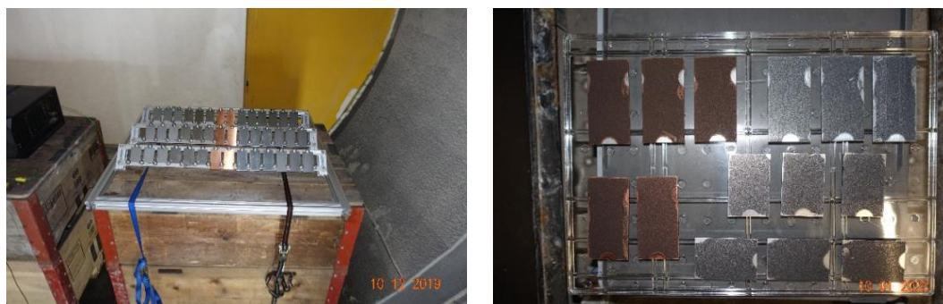
Figure 15 Corrosion monitoring in tunnel 'A'
