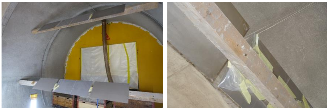
Figure 33 Climate monitoring in tunnels A (left) and B (right)
